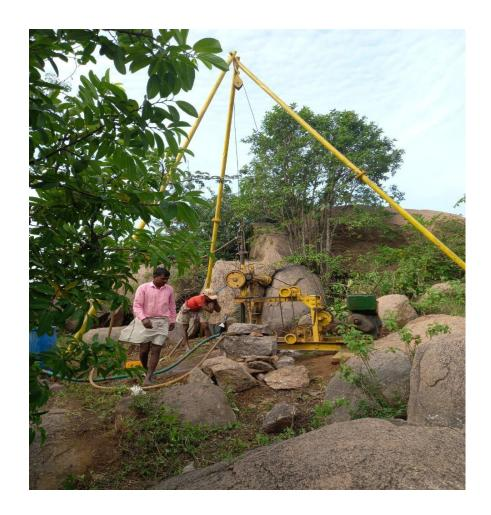
M/s. Adani (DC Development Hyderabad Ltd) is proposed to taking up the soil investigation work for **Proposed Data Center** HYD-21 at Shadnagar, Hyderabad, Telangana.
